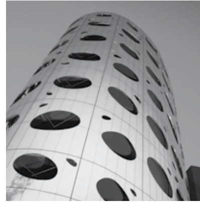
Futuristic architecture with an outer skin made of ALUCOBOND®: the Hotel Lindner Seepark in Klagenfurt, Austria
