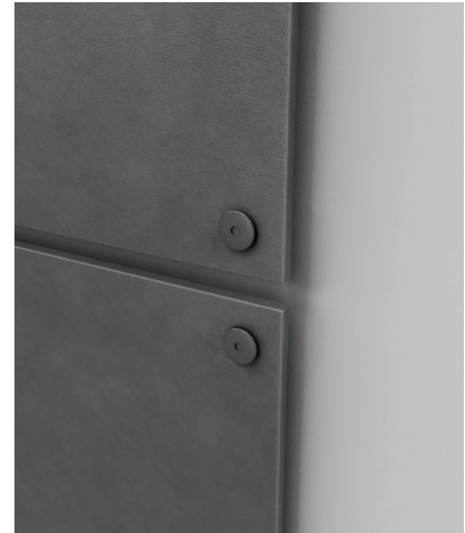
FIGURE 7 OPEN HORIZONTAL JOINT
