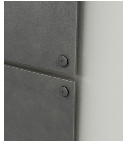
FIGURE 7 OPEN HORIZONTAL JOINT
